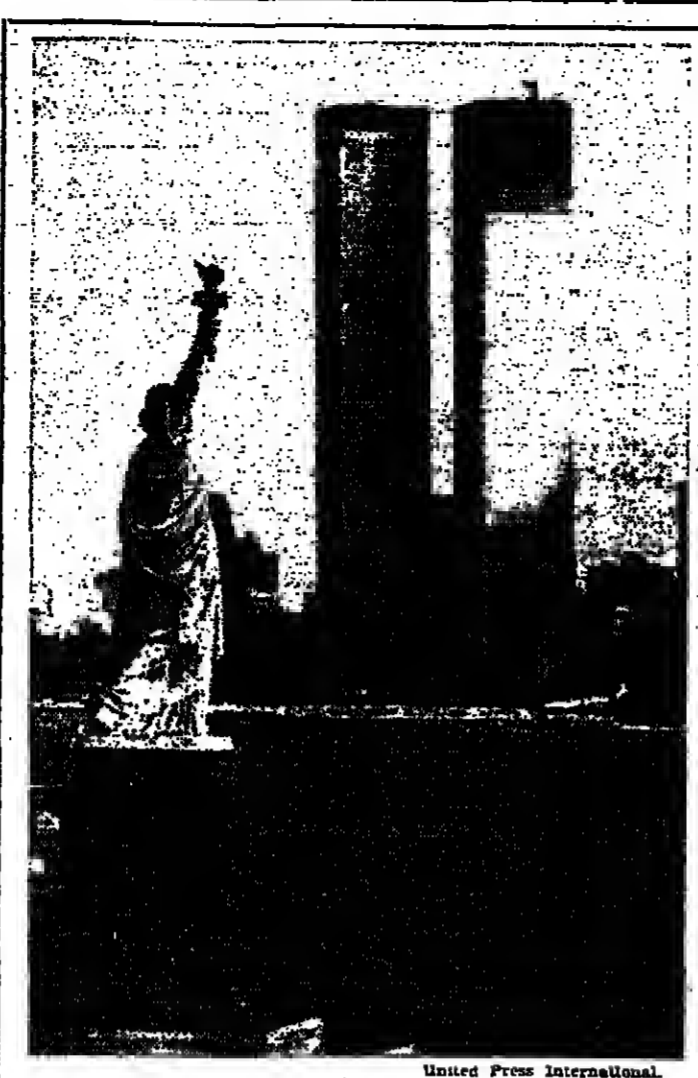
TALLER THAN TALL—With the Statue of Liberty looking on, work continues on New York's, and world's tallest building—the twin-towered World Trade Center, 110 stories (1,350 feet) high.
